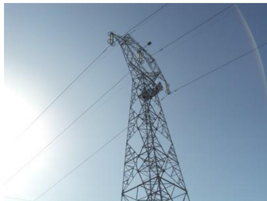
Figure 3. Temperature monitoring system of active conductor, type RITHERM [2].
