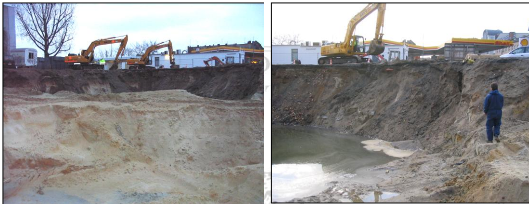
Fig. 2. Soil removal from the area of the former petrol depot at the former fuel station
