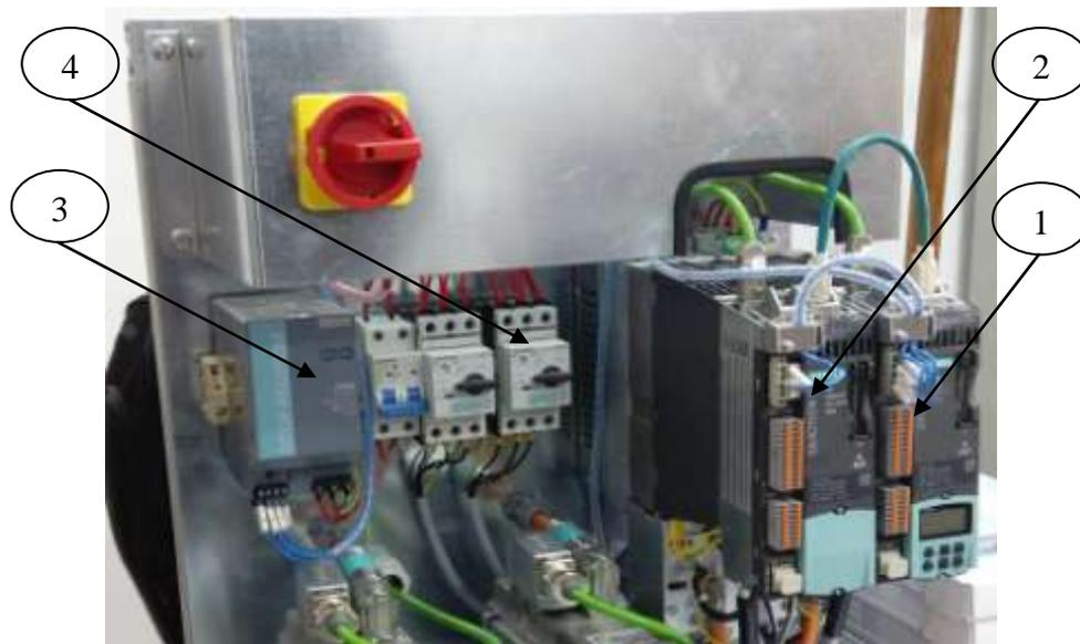
Fig. 2. The control equipment of the stand.
