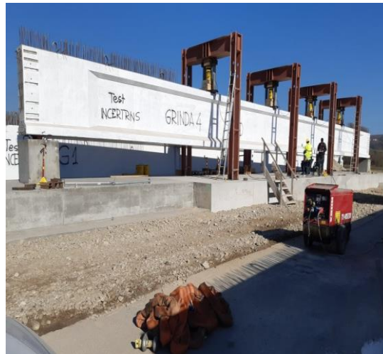
Fig 2. Location of the Beam and Hydraulic Presses on the Test Stand
