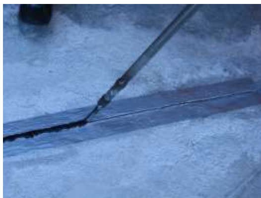
Fig. 2 Cutting asphalt to get a joint
