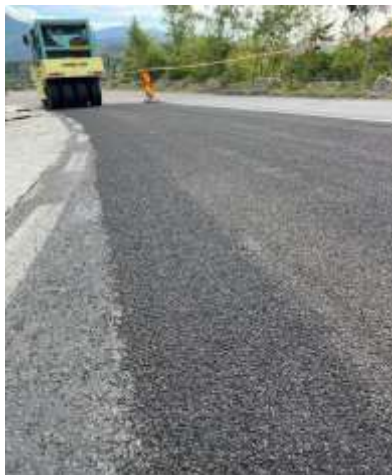
Fig. 5 & 6 Application of CARGOSFALT B product (basalt) on DN 73
