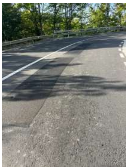
Fig. 7 DN 73 road arias treated with CRAGOSFALT B product (basalt)
