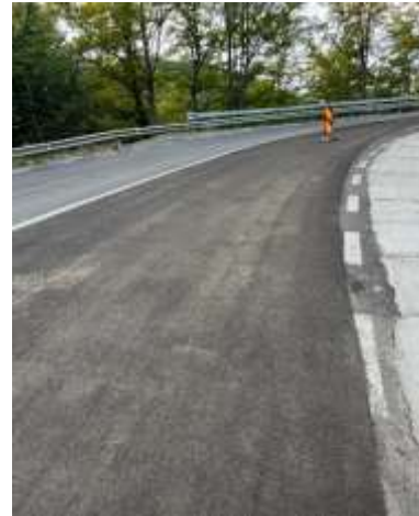
Fig. 5 & 6 Application of CARGOSFALT B product (basalt) on DN 73
