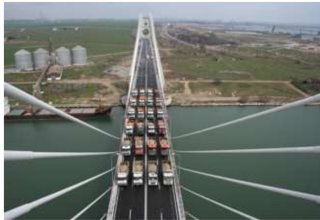
Fig. 2: An example of positioning of the test convoy [2]
