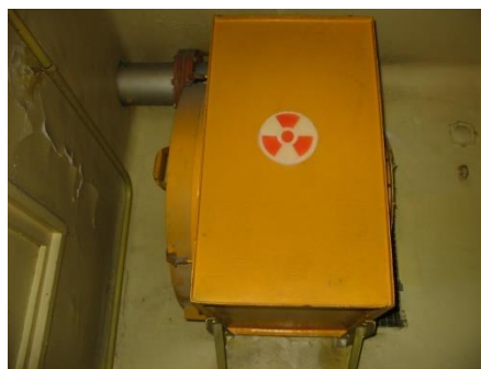
Fig. 2. HEPA ventilation system
