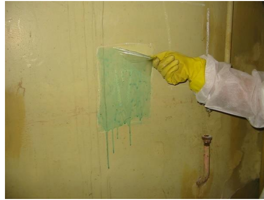
Fig 4. b. Wall decontamination
