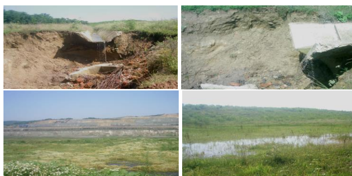
Fig. 16. Drainage channels destroyed the Bohorelu outdoor heap and accumulations of water at the base of the quarry
