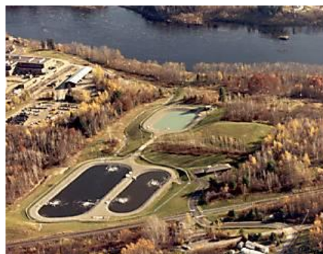
Fig. 8. – Sewage treatment lagoon in Germany
