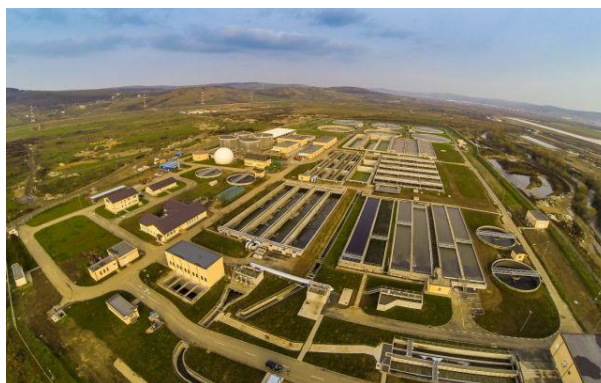
Fig. 1 – A complex wastewater purification station
