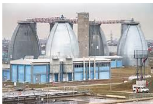
Fig.13. - Methantanks at the Bucharest purifying station
